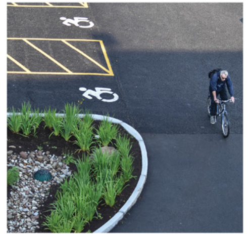
PERMEABLE ASPHALT AND CURBING
