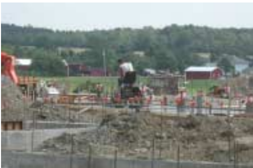
Finishing Cell Slab-HB
