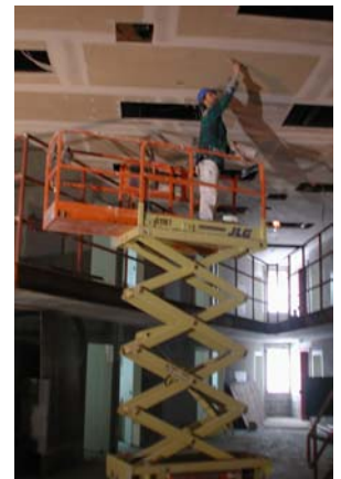
Ceiling work in HE:
