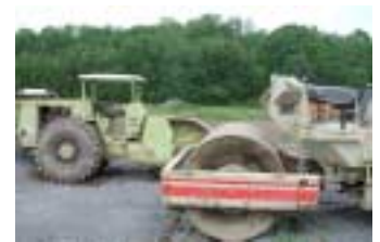
Rollers on site
