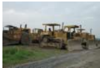
Bulldozers on site
