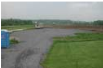
Construction Trailer Pad
