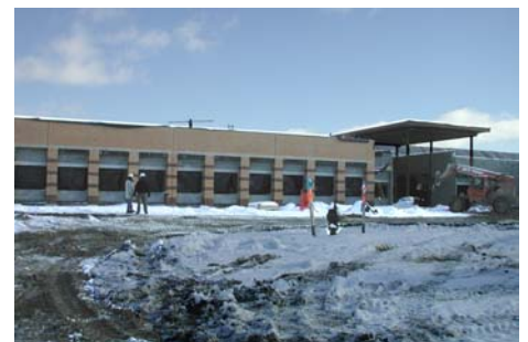
Exterior brick SB6
